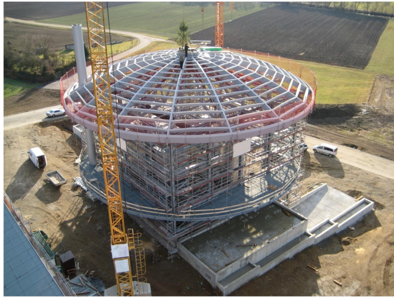
Main walls of biomass power plant in Schwendi
