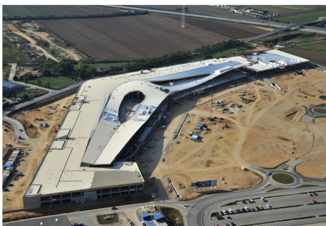
Aerial view of Shopping Resort Gerasdorf during construction
