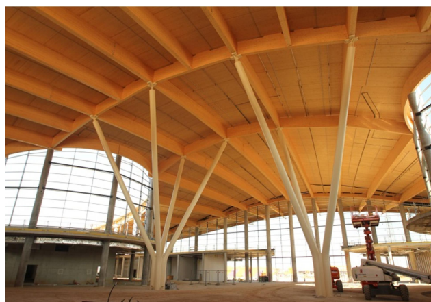
Interior view of roof construction consisting of timber (photos: ATP)
