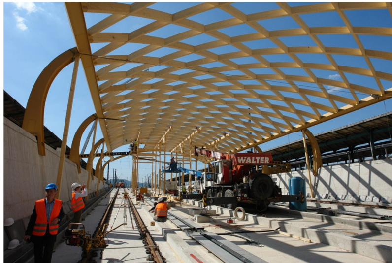
RegioTram station during construction phase (photo: osd)
