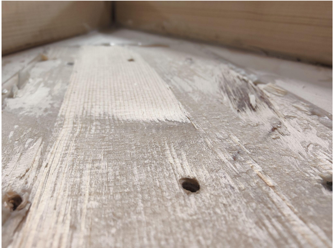
Figure A1.18.7 Glue-line failure at horizontal member
