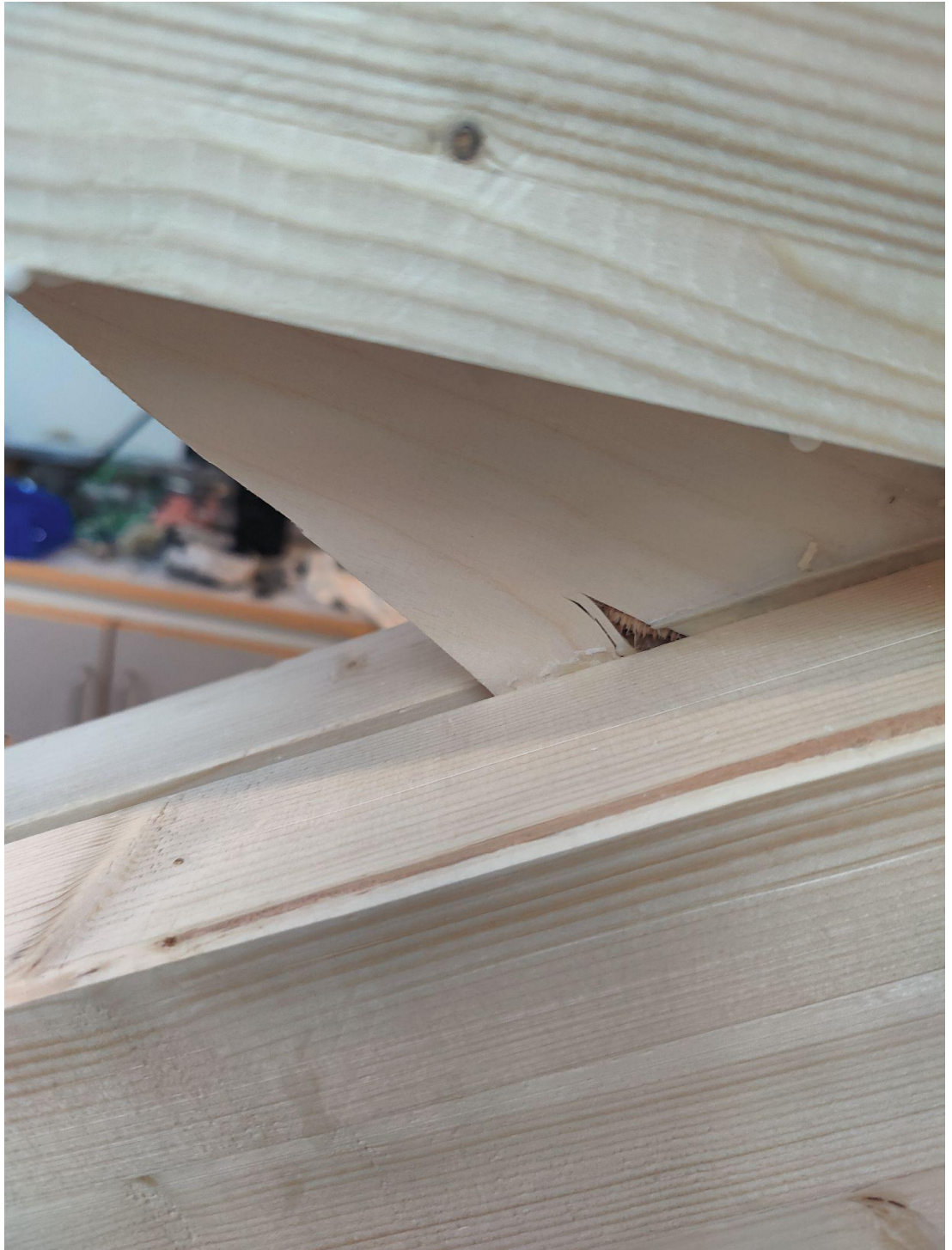
Figure A1.10.4 Small crack in plywood
