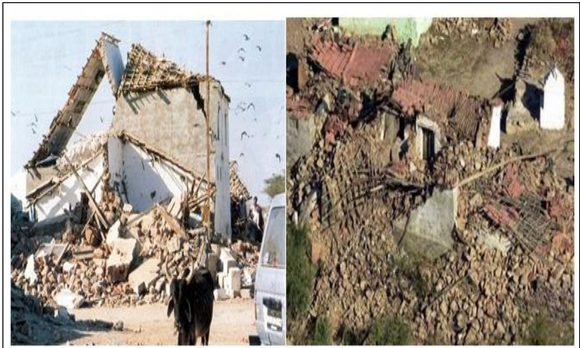
Figure 6.1 Bhuj earthquake damage to URM, 2001
