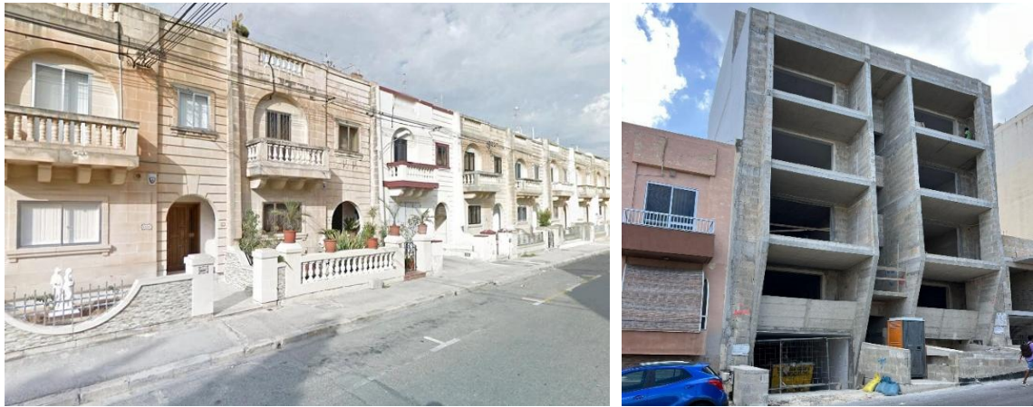
Figure 5:54 - Traditional terraced houses built using locally Globigerina limestone blocks, and modern apartment blocks built using locally Hollow Concrete Blocks (HCB) respectively
