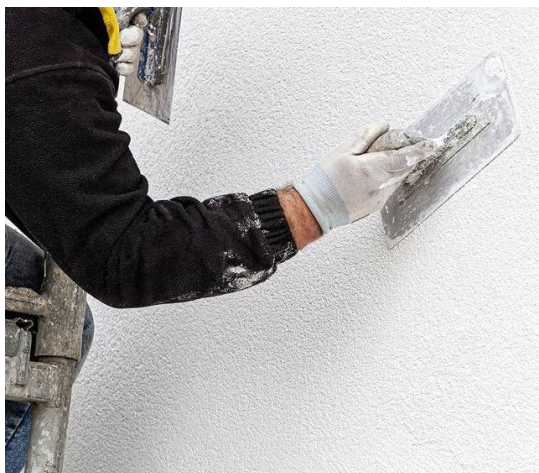
Figure 3:6 - Rendering of external masonry walls
