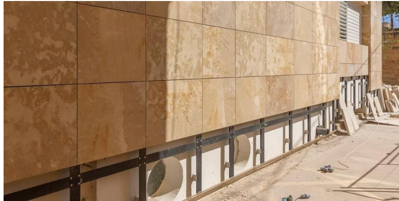
Figure 3:5 - Cladding systems supported by the masonry wall
