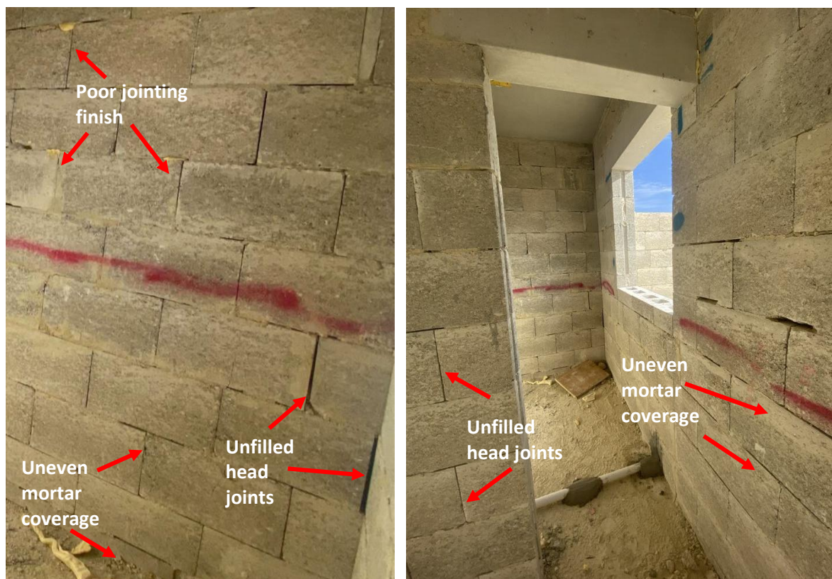
Figure 3:9 - Unfilled head joints, uneven mortar coverage & poor jointing finish
