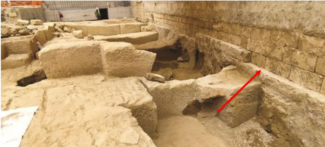
Figure 5:57 - Masonry walls constructed directly on the rock
