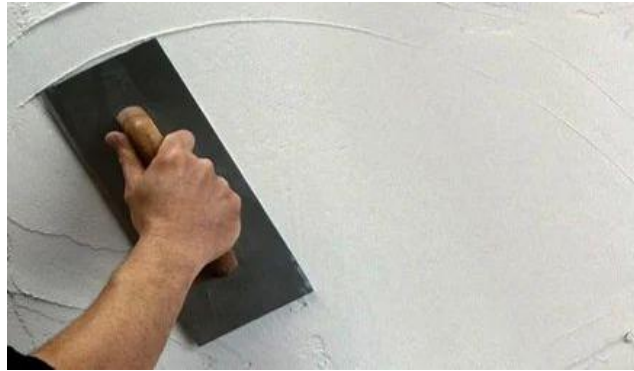
Figure 3:7 - Plastering of internal masonry walls
