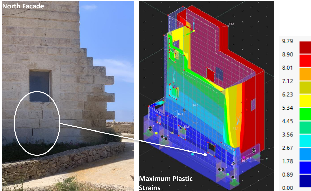
Figure 5:49 - Comparison between the numerical model and observed on-site cracking
