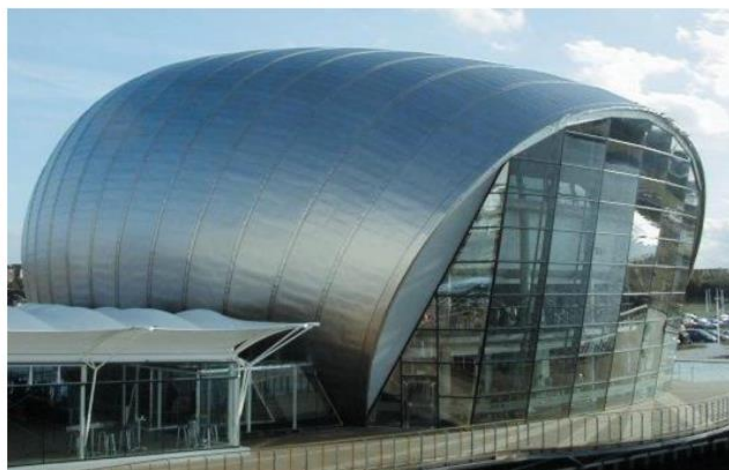
BDP Building Design Partnership: Glasgow Science Center, 3D Cinema, Glasgow, UK Project Execution: Mero GmbH & Co.KG
