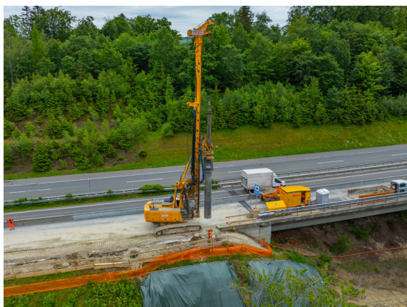
Figure 5 Chantier forage pieux D800
