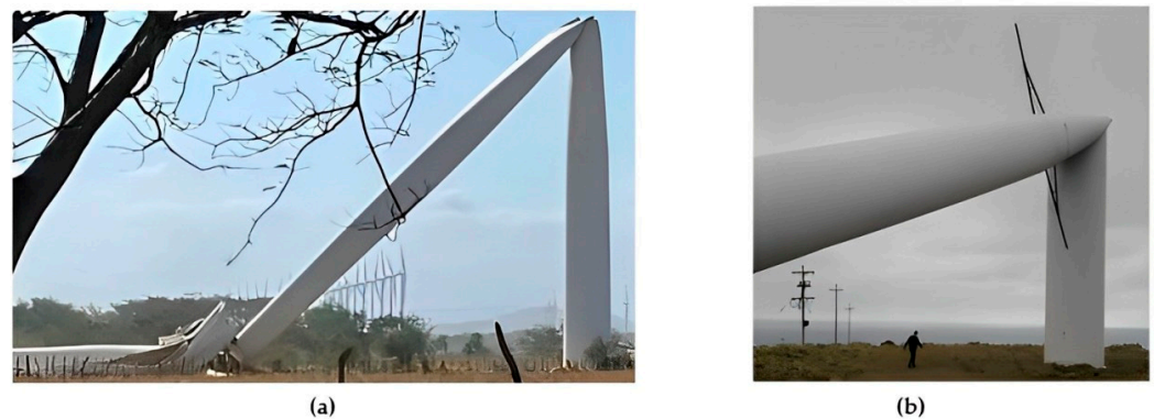
Figure 2. (a) Collapsed wind turbine tower in Maragatería, Spain [22]. (b) Collapsed wind turbine tower in Comodoro Rivadavia, Argentina [23].
