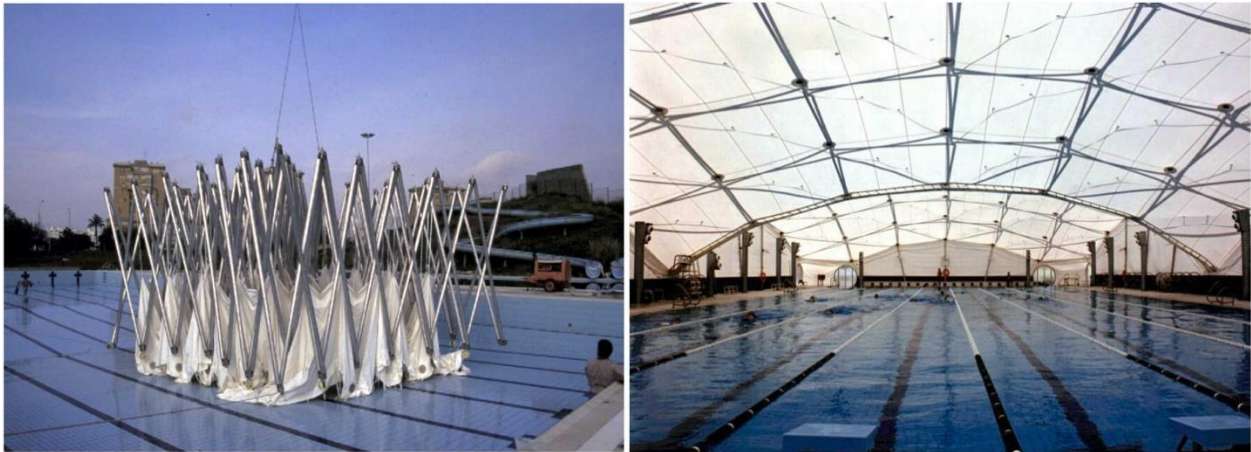
Figure 6. San Pablo retractable roof in Seville, Spain in its closed and open form [5].
