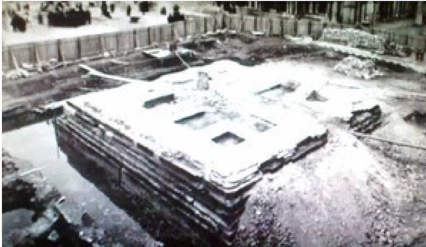
Figure 19. Foundation of the St Mark's bell tower after the collapse. (Umberto Sartori, 2012)
