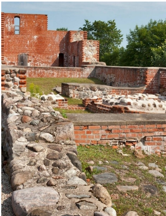
Figure 1. Turaida castle brick masonry walls with rubble stone core (Latvia) ( Alamy , n.d.)
