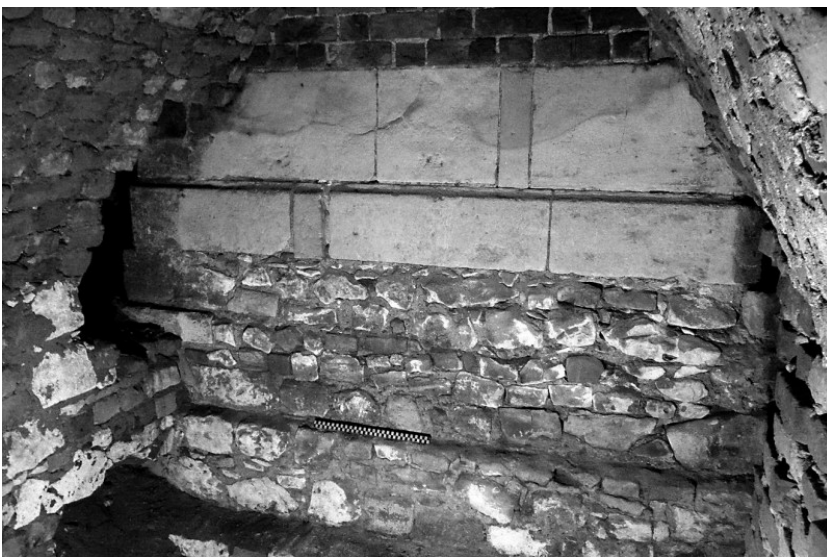
Figure 13. An example of a Gothic foundation in Poland (Saint Mary's Basilica). (Firlet, Kadłuczka, & Pianowski, 2011)
