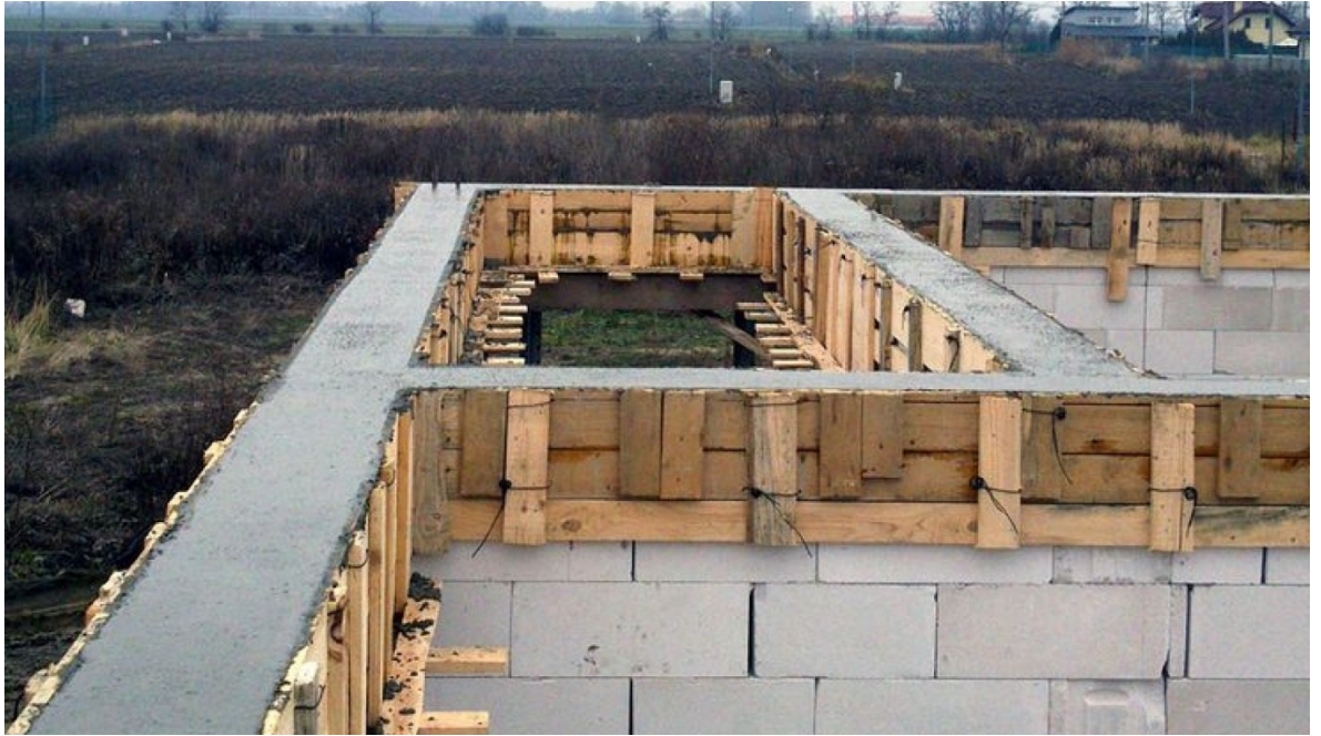
Figure 10. Ring beam (Taloasro, 2022)
