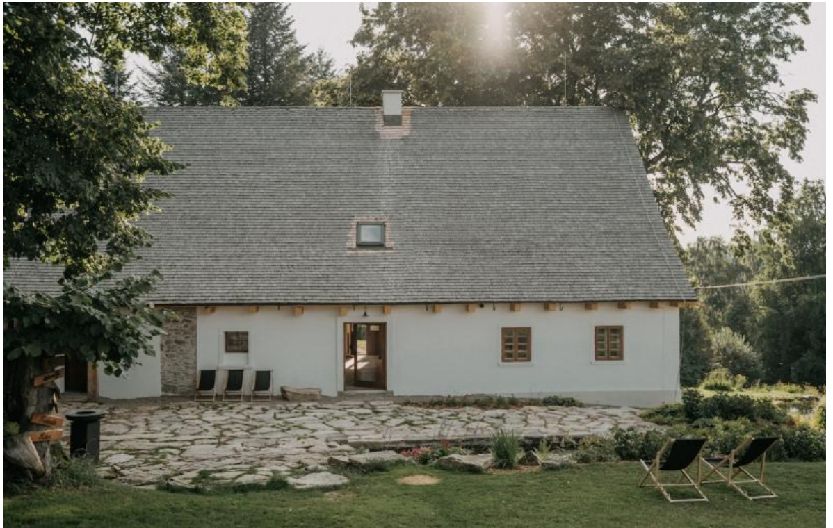
Figure 5. Typical traditional family house in Slovakia (Milliard City, 2022)
