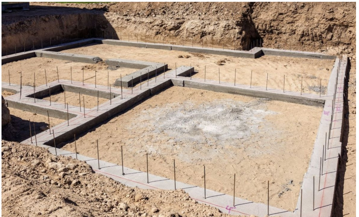
Figure 7. Building foundation (BMB Steel, 2024)
