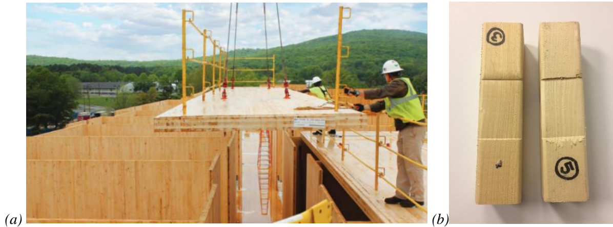
Figure 1-3: (a) Platform-type mass-timber building (Photo credit Lendlease); and (b) Compression perpendicular to the grain (Photo credit: Mpidi Bita)
