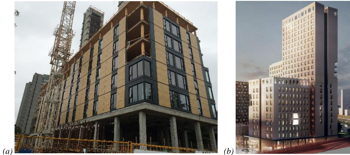
Figure 1-8: Hybrid construction: (a) Brock Commons (Photo credit Mpidi Bita); (b) and HoHo (Woschitz and Zotter, 2017) (Reprinted with permission)
