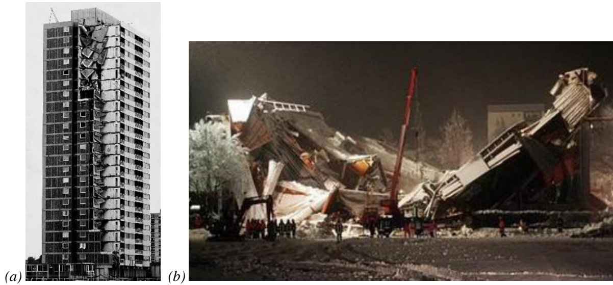
Figure 1-10: Disproportionate collapse incidents: (a) Ronan Point apartment (Macleod, 2014); and (b) Bad Reichenhall ice area (Winter and Kreuzinger, 2008)(Reprinted with permission)
